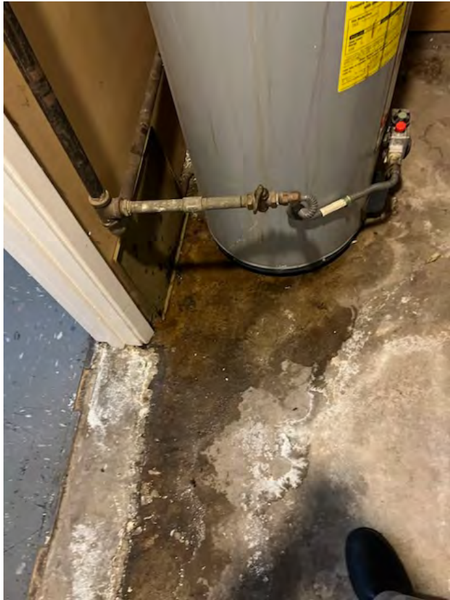
Water heater leak
