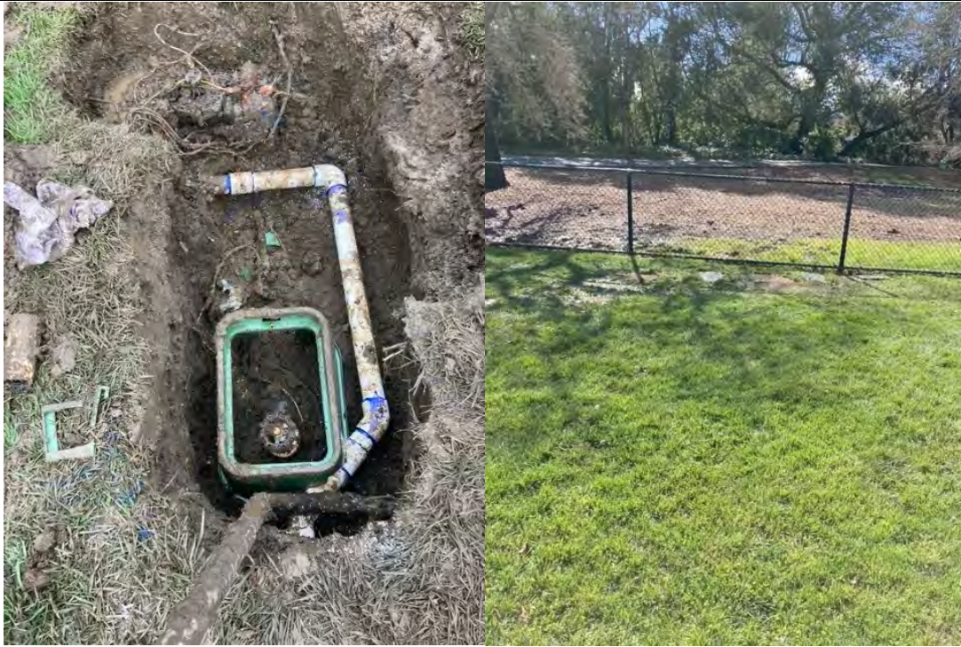
New gate valve installed
